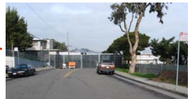
The Phase IA Construction fence is up!
